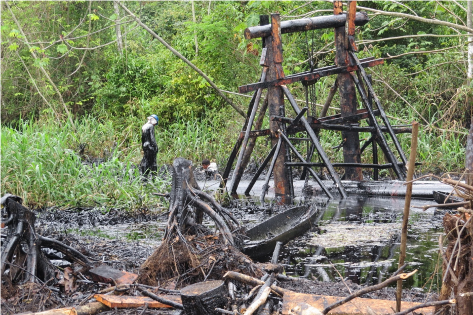
Photo 1: An indication of the pipeline's chronic state of disrepair and the impact that the Cuninico oil spill has had on the surrounding environment (Photo given to me by a Cuninico resident who himself received it from a Petroperu worker and used with their permission, June 2014).
